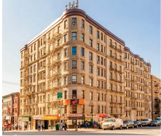
St. Nicholas Manor | Manhattan, NY | 112 units | Section 8
